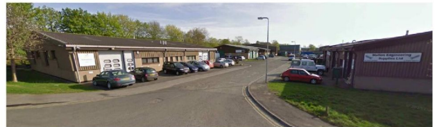
Use of industrial scale materials
