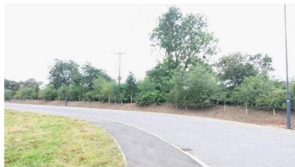
Western boundary of site, semi-established soft landscaping.
